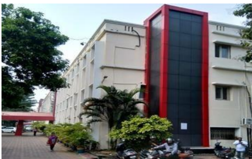
Figure 2 Secha Sadan building
